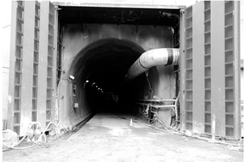
Caption: The entrance to the tunnel Picture – Ken Bell
